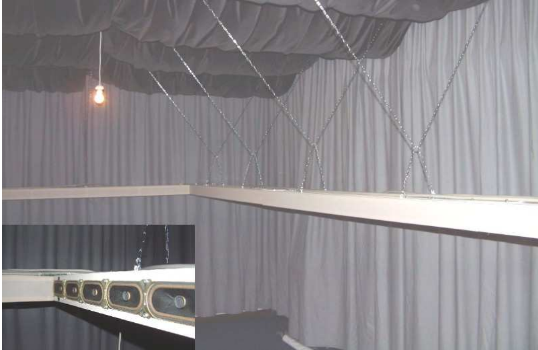
Figure 2.6 Speaker arrays for the TU Delft WFS system, set in: close up of the array.
